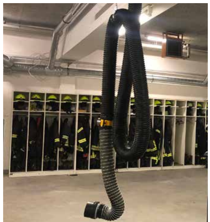
MRS installed in a fire station
