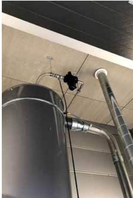
HVV Solo. Stand-alone side channel blower module.
