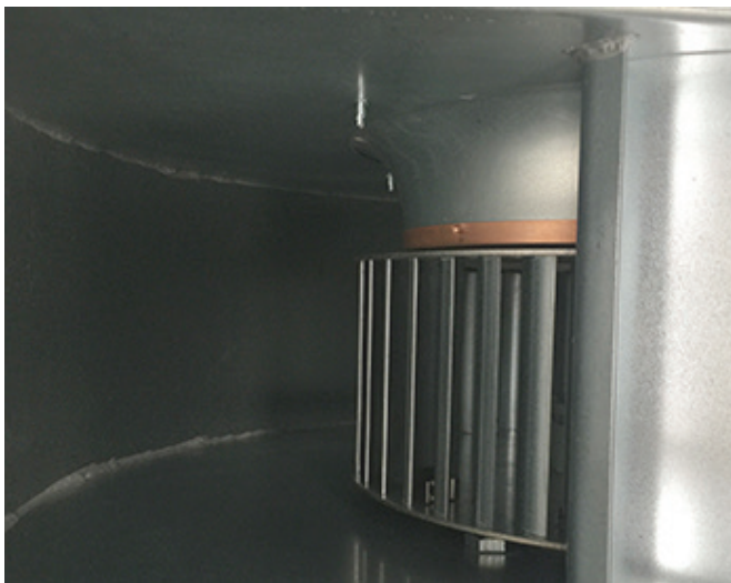
Example of spark protection on inlet (Copper ring)
