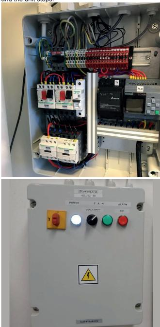
The electrical panel should be installed in an easily accessible and convenient place for the user and it must be connected 3 x 230 or 3 x 400V, 50 Hz.
