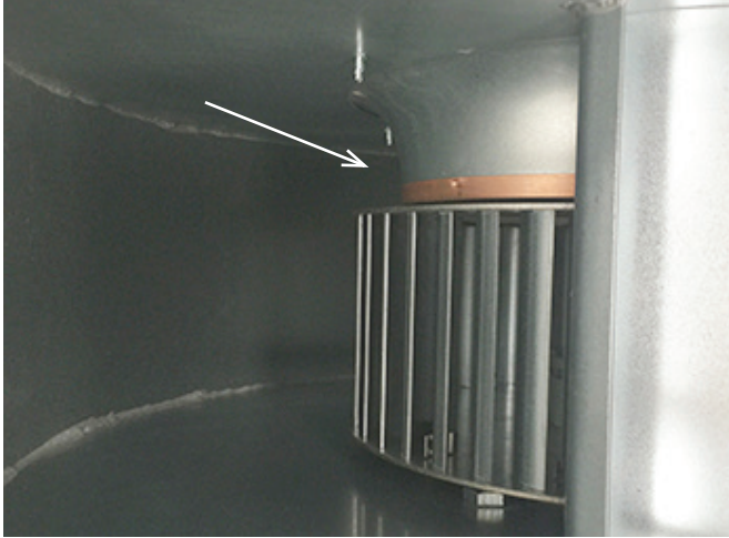
Example of spark protection on inlet (Copper ring)
