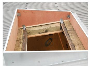
For directly mounted diffuser solution, the hole in the roof must be  $1160 \times 820$  mm.
